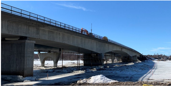
Figure 19. Kalix bridge picture.
